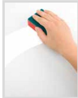
Surfaces need to be clean, dry and free of grease. Depending on the material, remove all rust, apply filler, sand and clean. Cover all surfaces that are not to be painted with paper and tape, then prime the surfaces.
